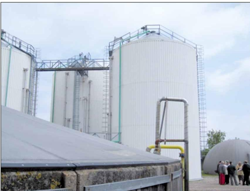
**Figure 2:** Vertical steel tanks for the digestion of mixed wastes from agriculture and industry in Denmark
