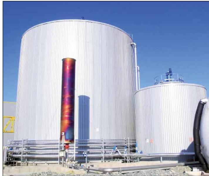
**Figure 8:** Industrial design of a waste digester with (from right to left) gas balloon, pre-acidification tank and digester. (Picture courtesy of BDI).
