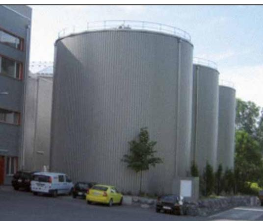
**Figure 14:** Digestion of expired food from distributors and rendering waste (Bösch Brothers, Switzerland)
