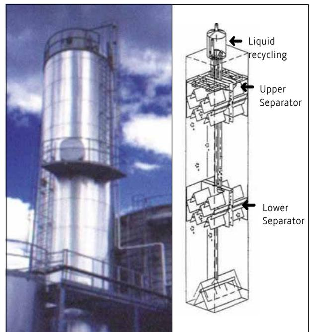
**Figure 7:** EGSB Dairy waste water treatment with internal circulation, Emmi, Switzerland
