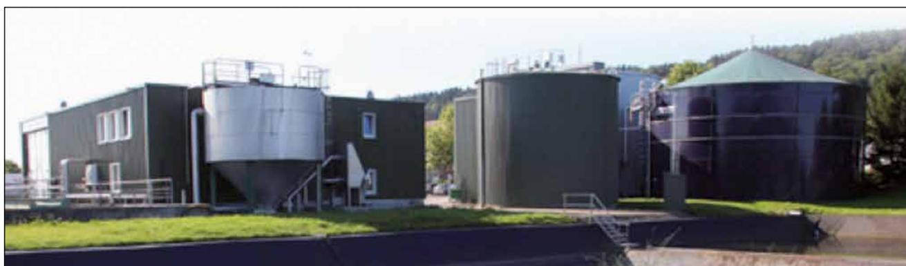
**Figure 4:** Digestion of vegetable waste in a contact reactor: Gastro Star, Switzerland (Forster AG)
