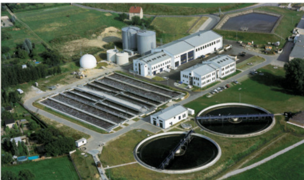
Co-fermentation plant Radeberg (source: Strabag 2013)
