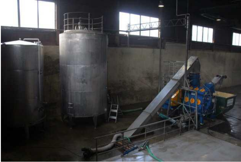
Hammer mill and storage tanks (picture Abwasserverband Zirl)
