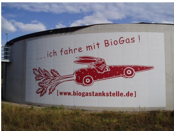
Biogas plant and bio-methane filling station, Dannenberg
